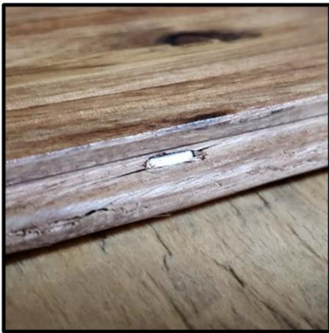
Cleat properly driven and no splitting
