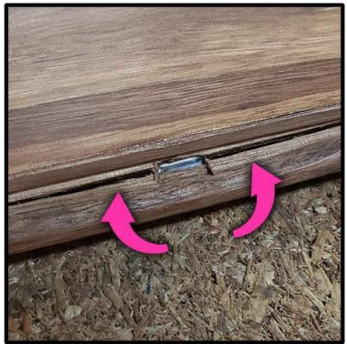
Cleat properly driven and some splitting
